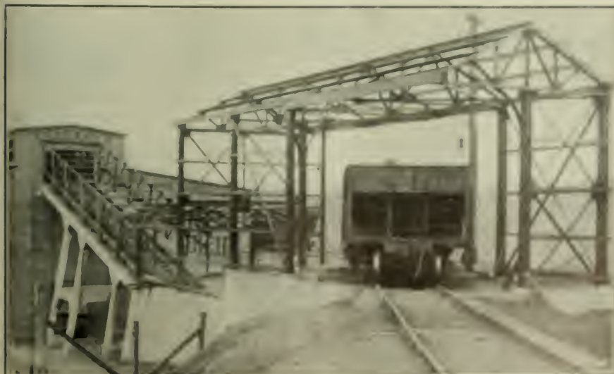
FIG. 6 SHOWING THE COAL CHUTES INSTALLATION
